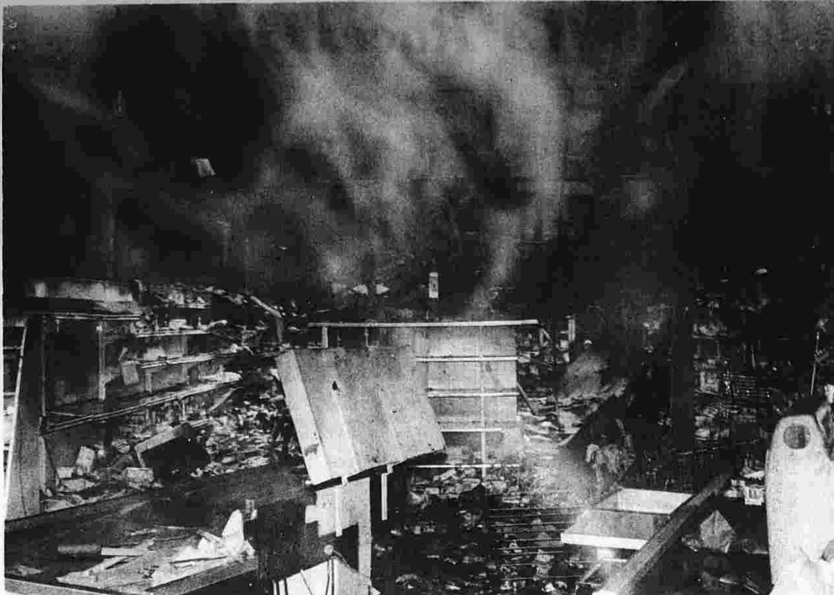
The ceiling of the IGA Foodline Market at Vernon Circle hangs precariously over twisted shelves which were once piled with food items all destroyed in a Saturday night fire of undetermined origin. (Herald photo by Richmond)
